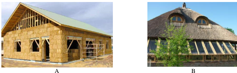
Figure 5. Building construction with straw bale load bearing walls (Adam and Ali 2015) -A, Newly built straw house of the Đupovac family (Šabac) (Aleksić gradnja, 2018)-B.
