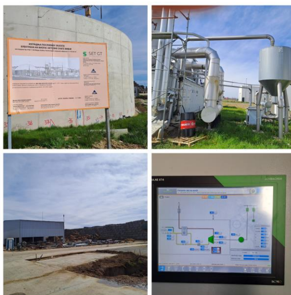
Figure 3. Biogas plant SET Green Technology.
