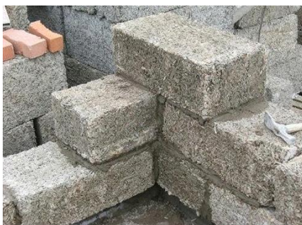
Figure 8. Straw concrete blocks (sand and gravel+ cement+straw).
