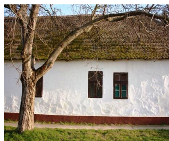
Figure 4. Old houses built with “charges (naboj)” from Mošarin, Serbia.
