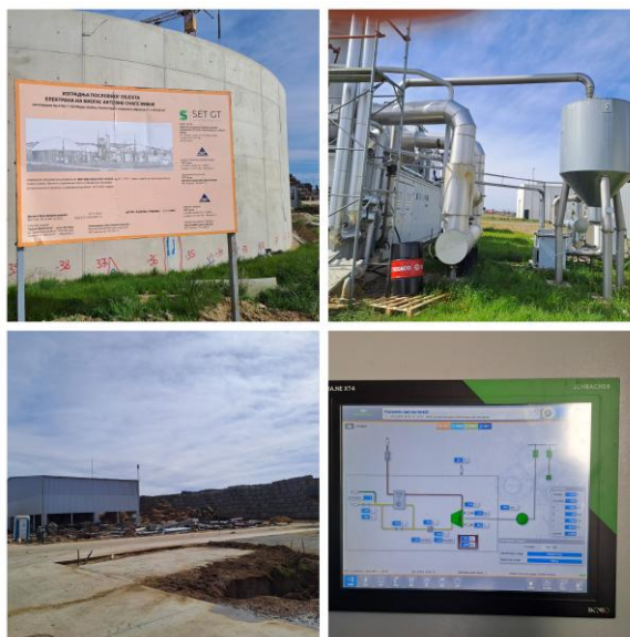
Figure 3. Biogas plant SET Green Technology.
