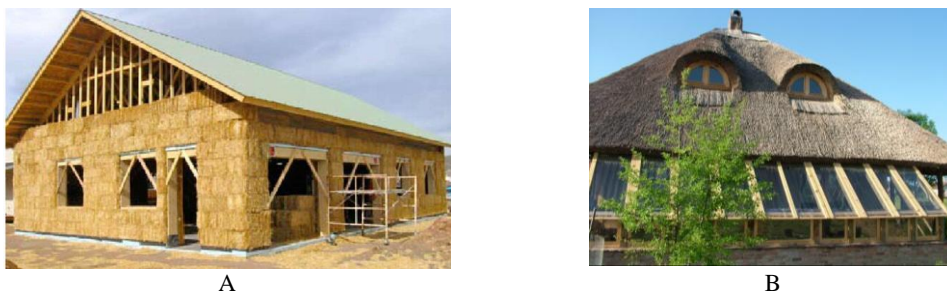
Figure 5. Building construction with straw bale load bearing walls (Adam and Ali 2015) -A, Newly built straw house of the Đupovac family (Šabac) (Aleksić gradnja, 2018)-B.
